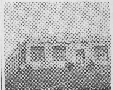
New Plant Now Overlooking Jon Falls Expressway
